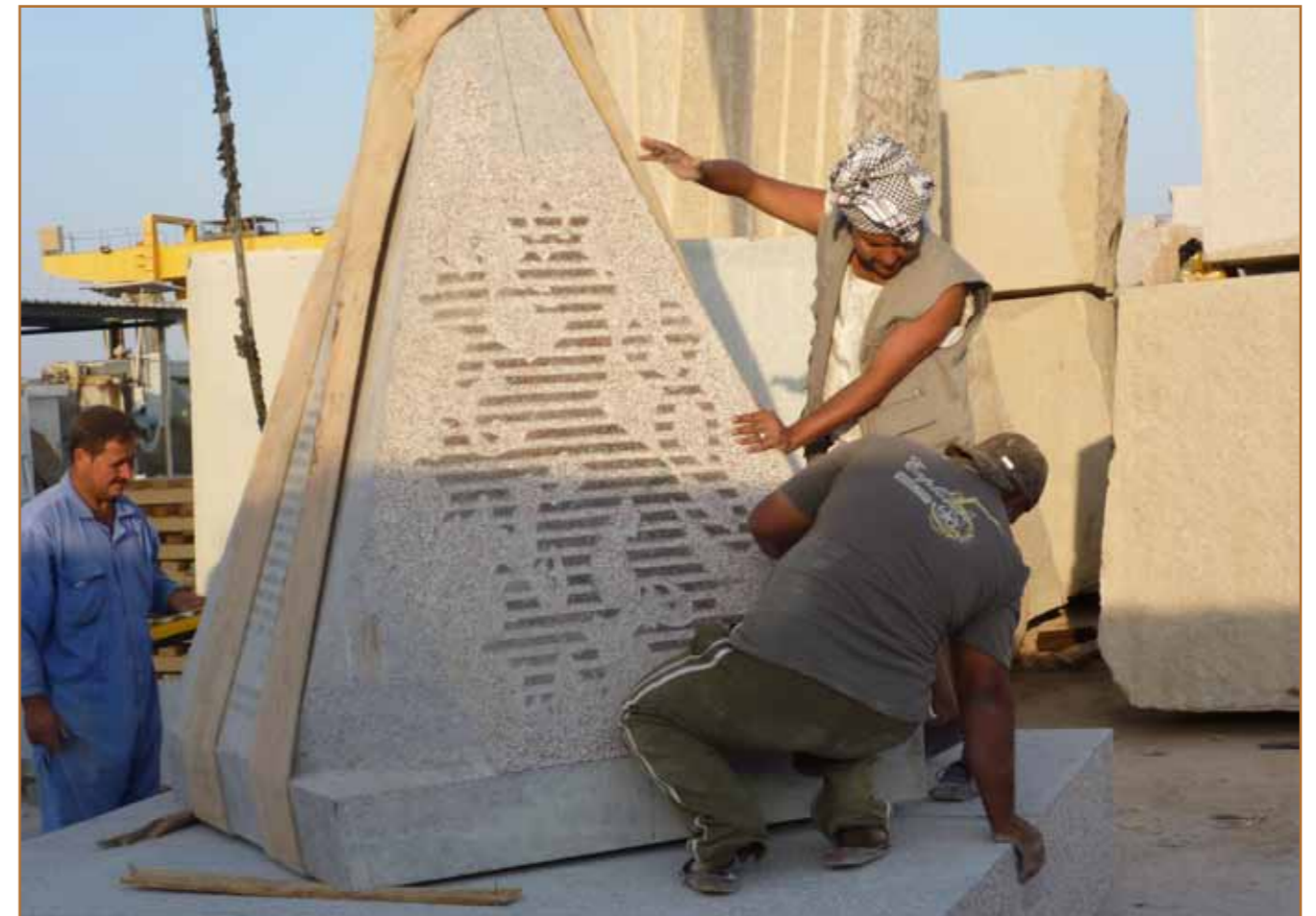
Final assembling of all parts together (Workshop in Aswan)
