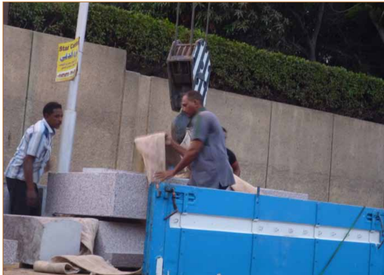
Instalation works in progress (Cairo)
