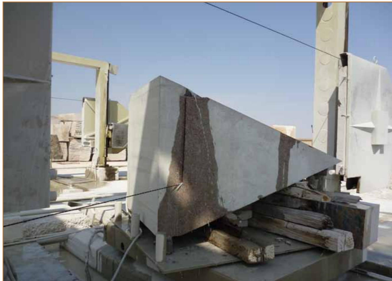
Cuting in progress (Workshop in Aswan)
