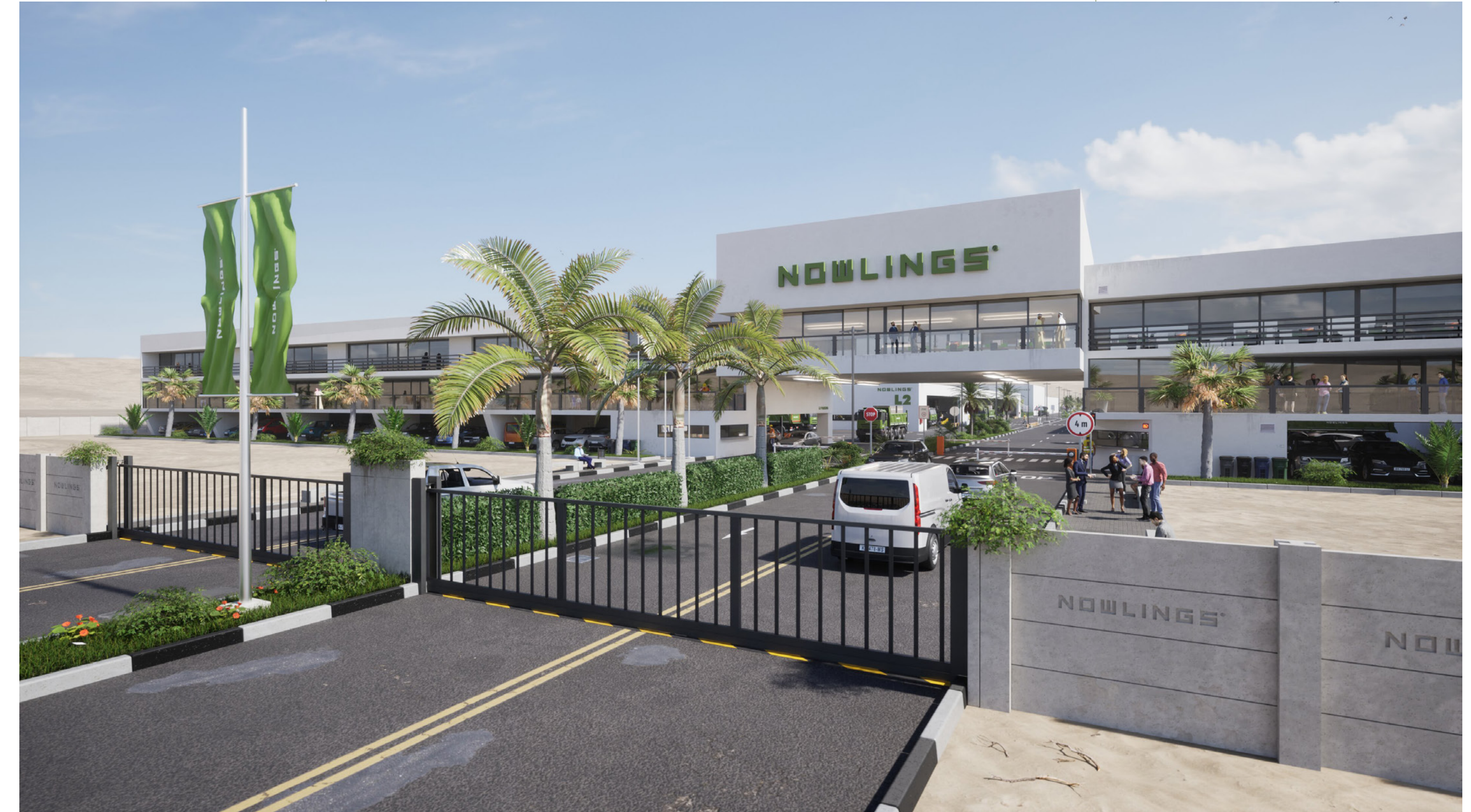
Entrance / Gate and Offices
