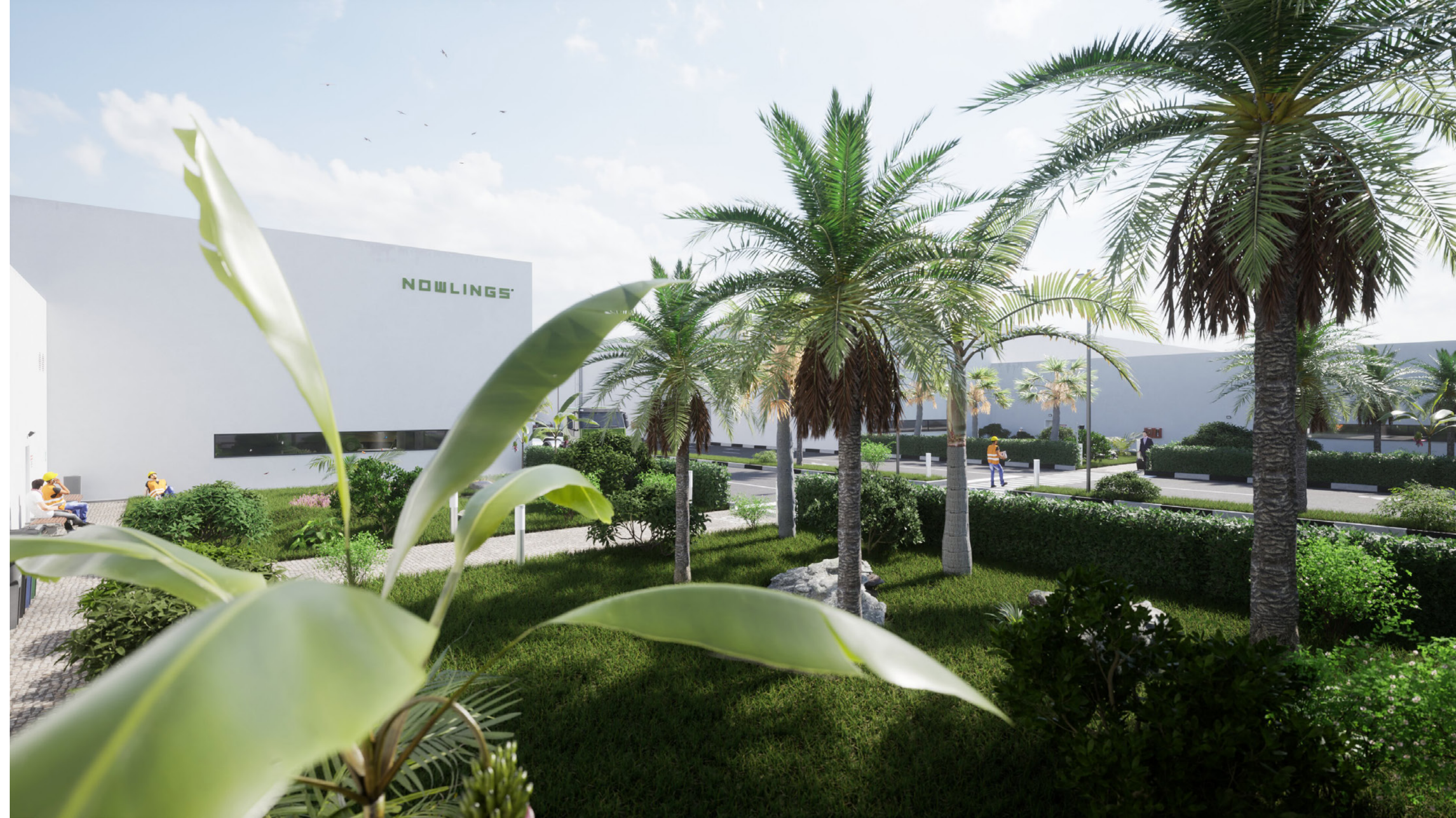
LINE 2 - Relaxing green zone, front of Curing station hall, behind: Board production hall 2
