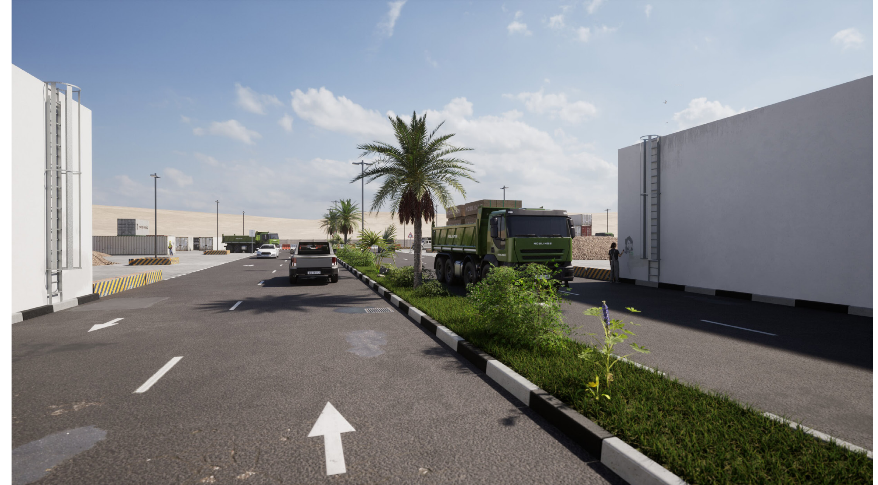
Approaching concrete reinforced Open areas front of Wood preparation halls LINE 1, 2
