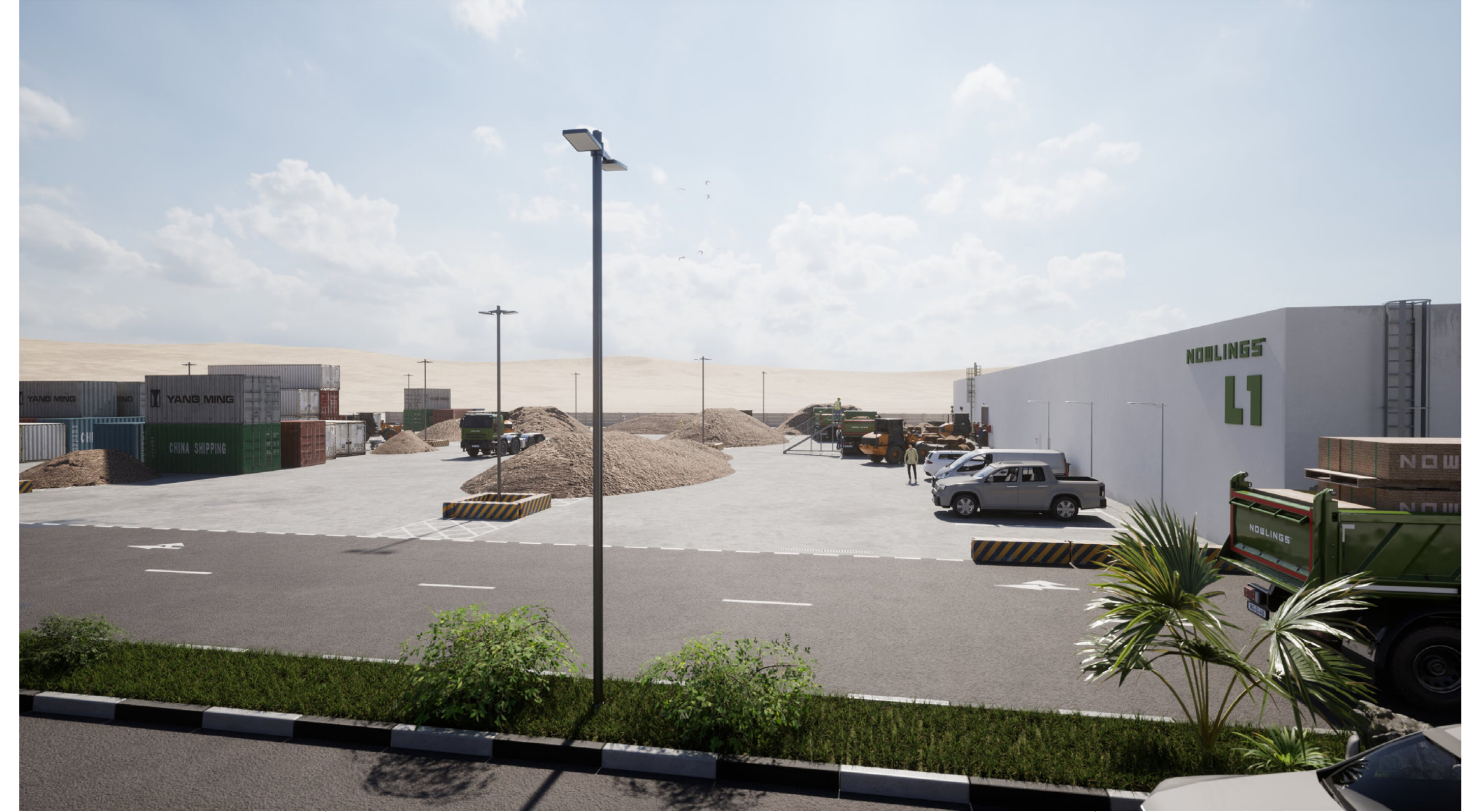
LINE 1 - concrete reinforced Open area
